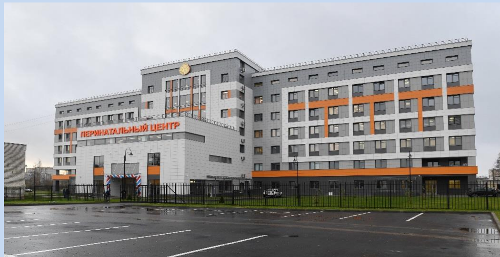
State Budgetary Healthcare Facility of LO “Interregional clinical hospital of Gatchina” (Perinatal center)
